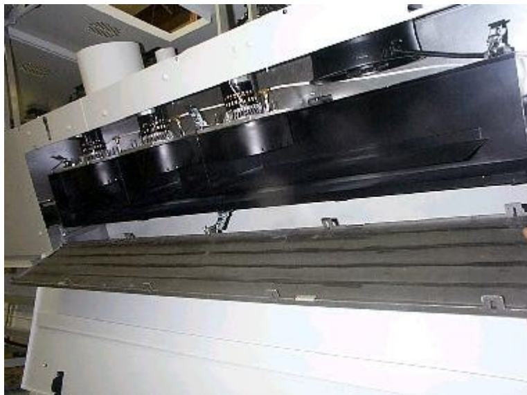
Access To Flux Separation Box For Routing Maintenance Photo 2
